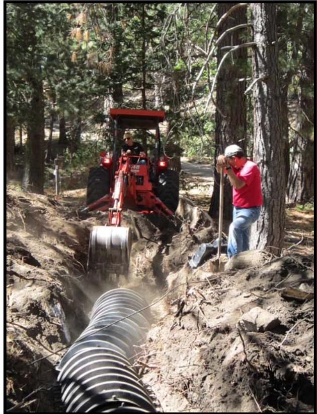
*Digging the trench and putting in the new drain field for Lolomi Lodge*
